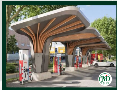
MDI EV CHARGING STATION
